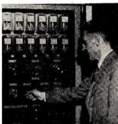
WOW-TV Omaha Chief Engineer Bill Kotera turns switch sending station's power to 28 kw from 17.2 kw previously authorized, after quick FCC decisions two days apart, first authorizing station 28 kw and then 100 kw. Station expects to increase power to authorized 100 kw during January, when it receives additional technical equipment.
